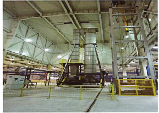
立式淬火炉 Vertical type quenching furnace
